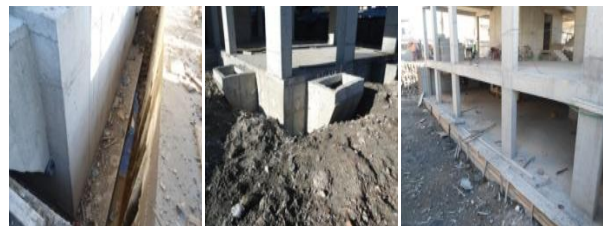
Figure. 3.2.1: The foundation of the project.
